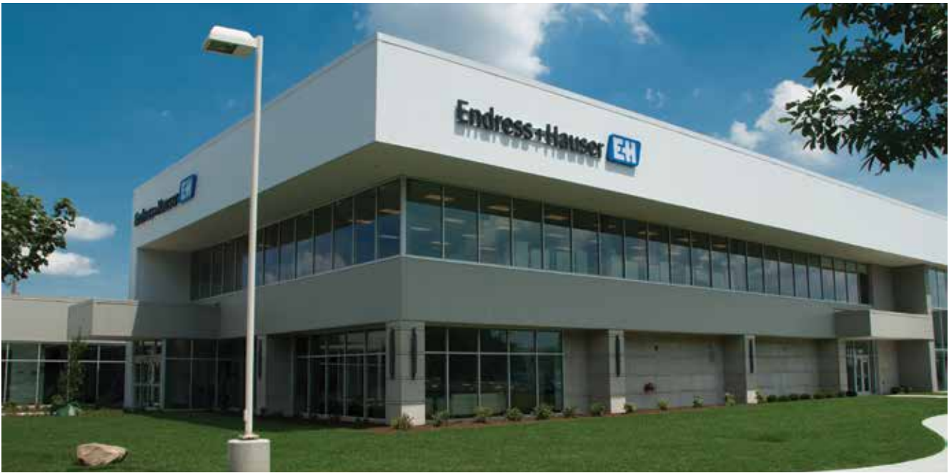
Endress+Hauser Customer Center, Greenwood, IN
