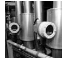
Flowmeters mounted in a fluid riser vertical pipe
