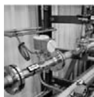
t-mass measuring nitrogen consumption
