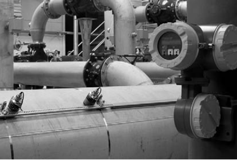
Standard horizontal installation of a clamp-on device
