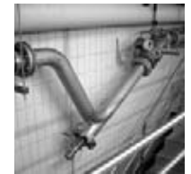
EMF mounted in a siphon
