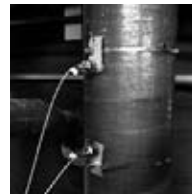
Installation on coated pipes
