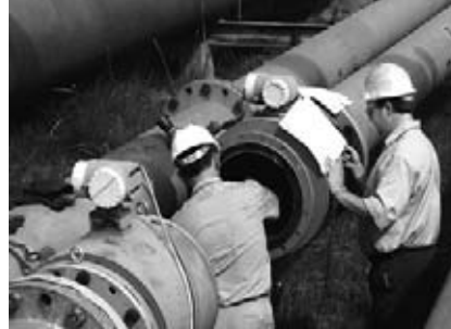
Inspection of the flowmeter pipe
