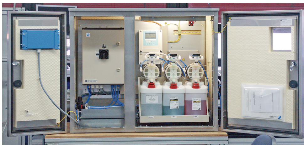
CYC310 system in stainless steel cabinet, includes CPC310, buffer solutions, pumps, transmitter and display unit.
