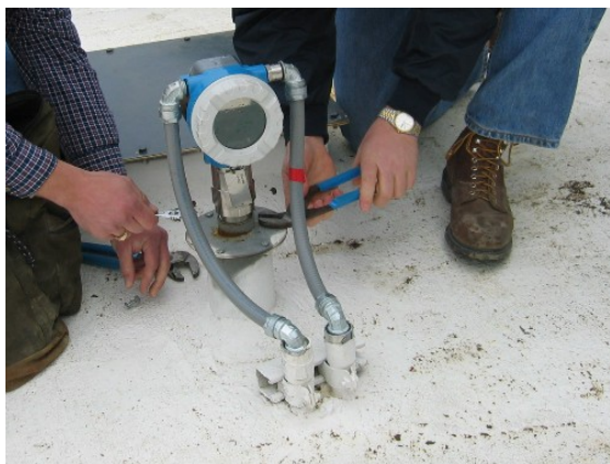
Levelflex M - FMP40 installed on top of 125ft high silo
