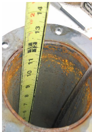
Levelflex M - FMP40 installed in nozzle (12" tall, 4" diameter)
