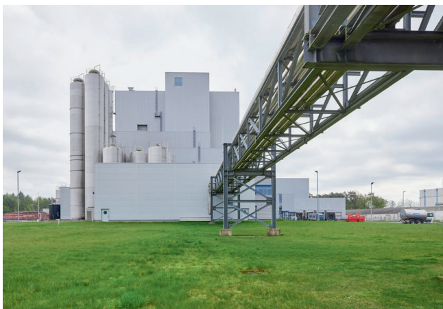
New spray drying facility at the DMK Group location in Zeven.
