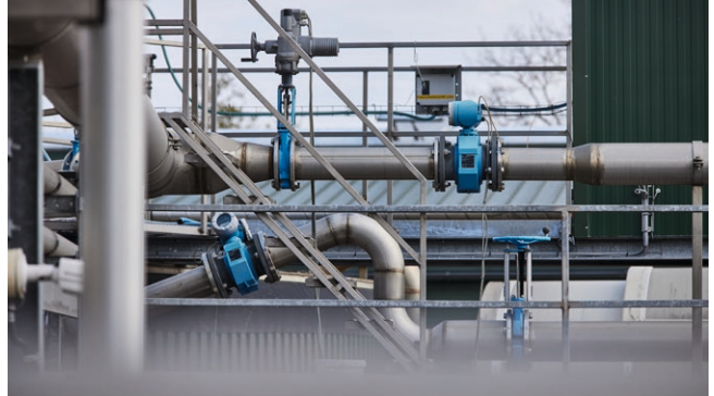
Proline Promag P: the robust electromagnetic flowmeter for demanding wastewater applications.
