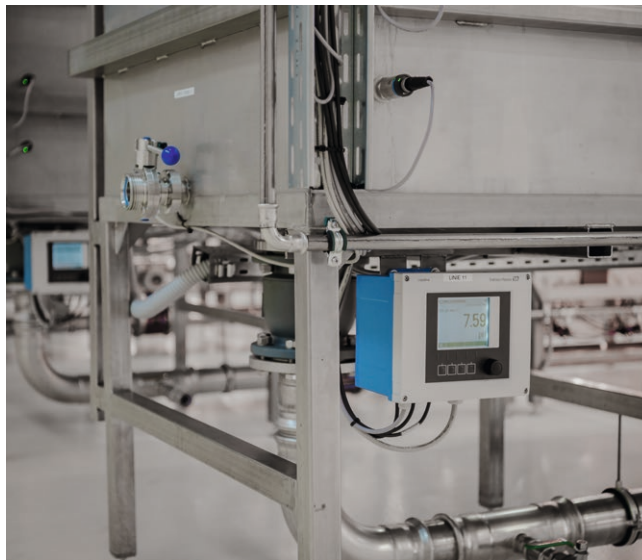
The Liquiline CM444 transmitter collects the pH, conductivity, and turbidity values.
