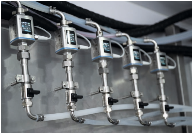
Picomag with a nominal diameter of DN 15 for monitoring the volume of non-alcoholic beverages from the keg.
