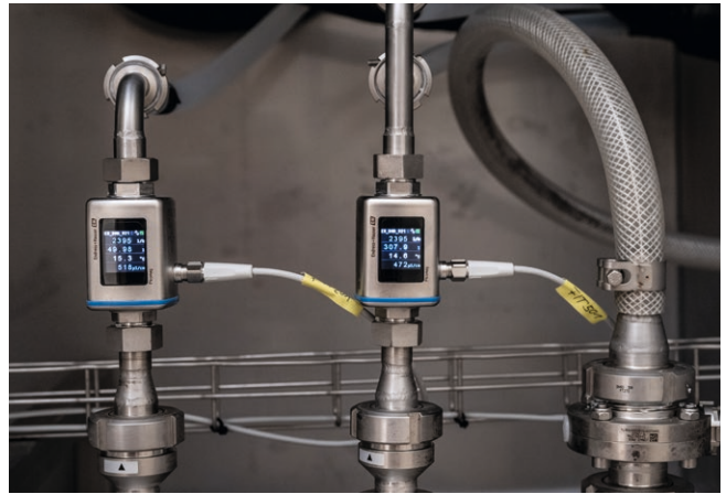
Jack-of-all-trades. The Picomag simultaneously monitors flow, temperature and conductivity.
