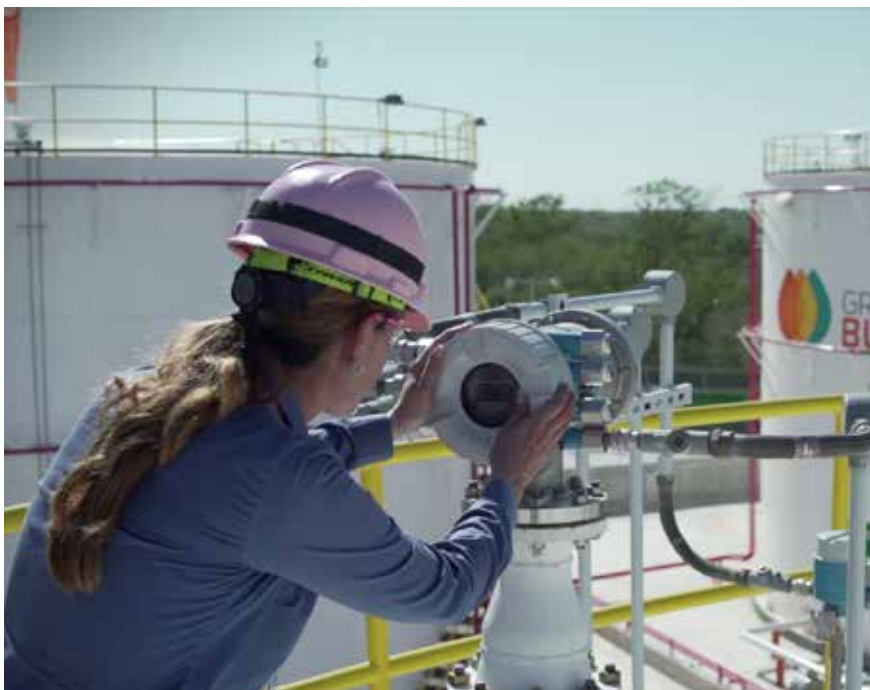
Servo tank gauging instruments offer high precision measurement.
