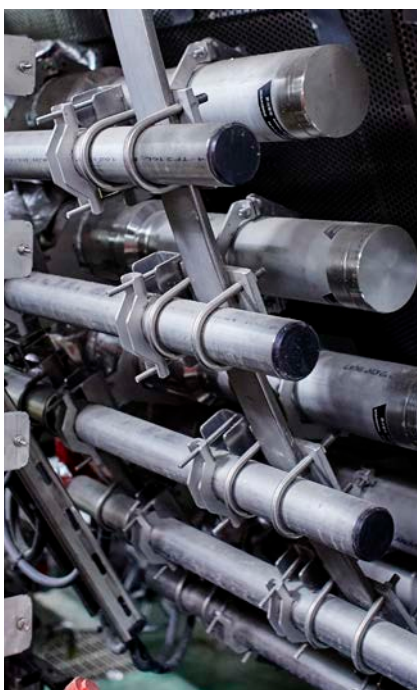
Arrangement of detectors for the profiler system on the tank.
